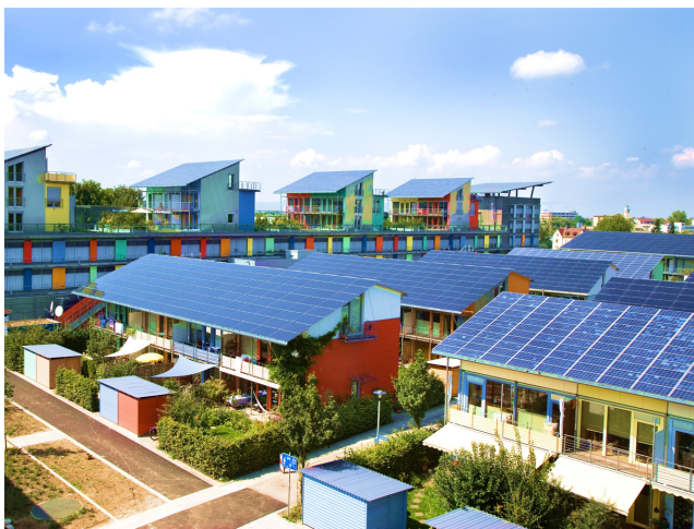
Figure 6 | Distributed energy sources powering The Solar Settlement in Freiburg, Germany. This community produces 300 percent more energy than it requires to operate. The sale of excess energy back to the grid generates annual profits of $5000 per household. Image from Wikipedia.org (2016).
